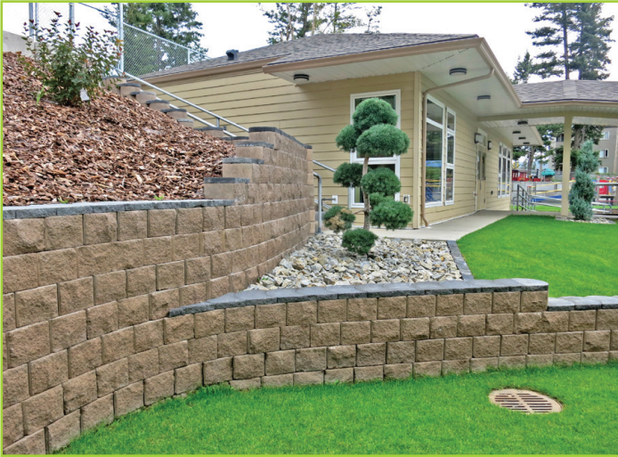
ROCK FACE WALL WITH TERRACES
