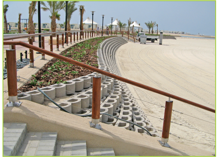
CURVED ROUND FACE RETAINING WALL
