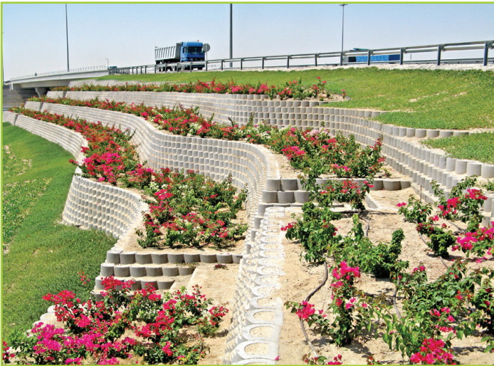
ROUND FACE TERRACES AT AN INTERCHANGE
