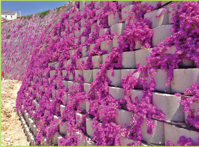
PLANTED ROUND FACE RETAINING WALL
