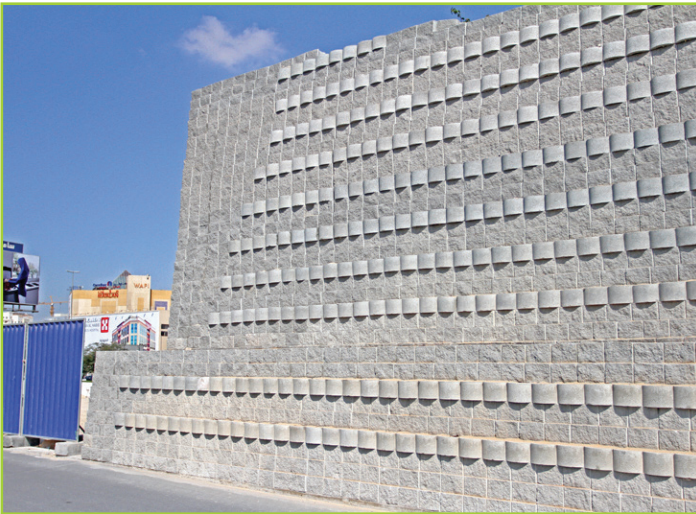
SOUND BARRIER WITH ALTERNATING FINISH
