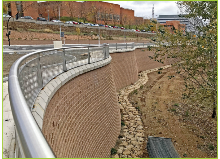
CURVED WALL, SUPPORTING HIGHWAY
